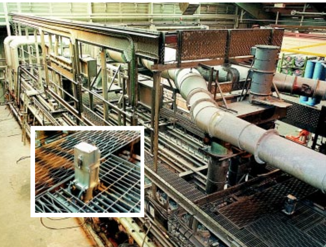
Photograph shows installation on a pattern glass plant
