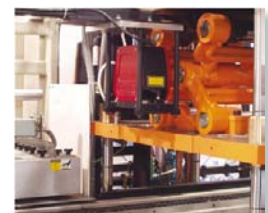
Typical LSP installation
